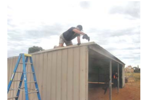
Brian Marshall putting flashing on
